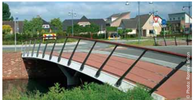
Fixing of bridge railings
