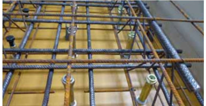
Installation of fixing anchors
