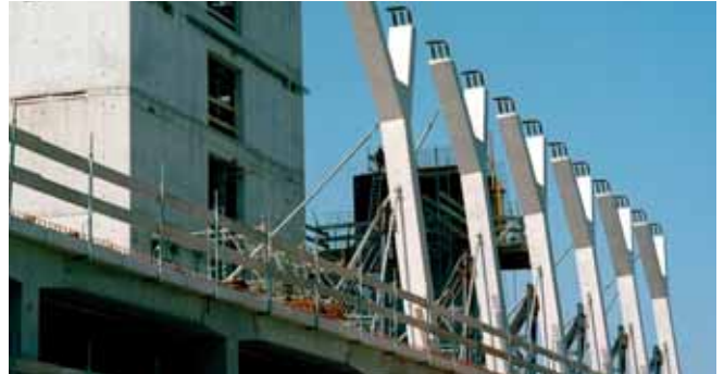
Fixing and adjusting precast elements
