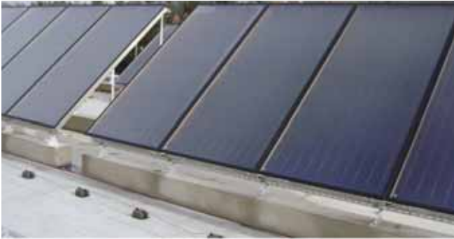
Fixing of solar panels
