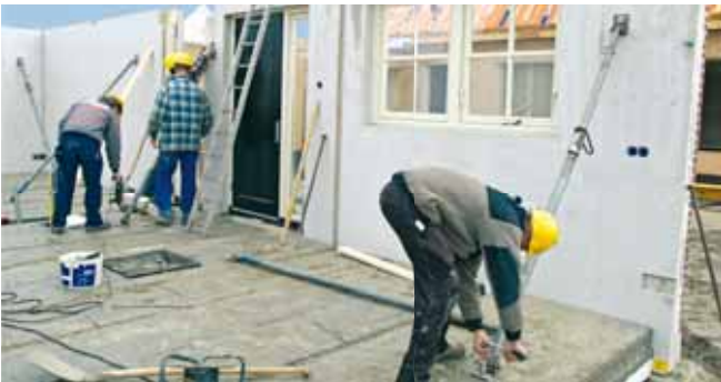
Fixing props to precast elements
