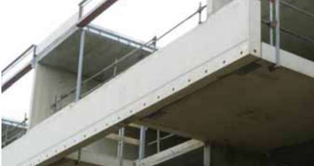
Fixing of balcony railings
