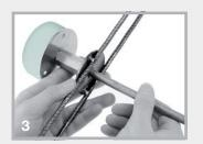
Screw axis through the fixing spider and fasten fixed earthing terminal
