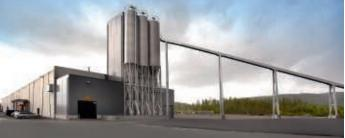
Tower plant with 2 – 2250 litres mixers for production of railway sleepers.
