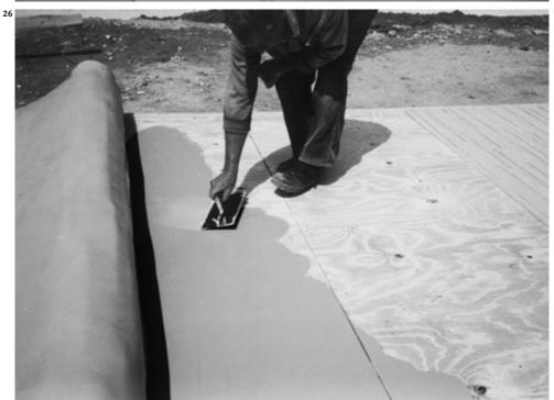
and roll it up again on to the 'transport jacket' (cardboard roll) making sure that formliner is in the right position to be rolled out onto the Formliner Adhesive and shutter. The use of the stripping jackets will make it easier to move the formliners around the working area.
