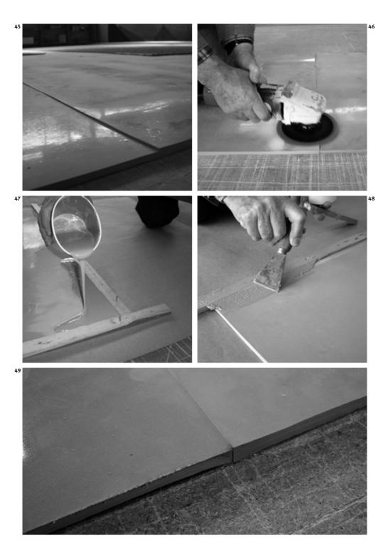
**Note:** To extend the workable time of Elasto Filler spread the mixed filler onto a board as a thin coat.
