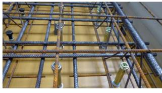
**INSTALLATION OF FIXING ANCHORS**
